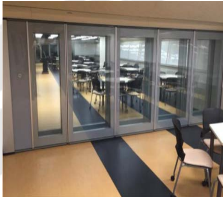
Fig. 4 Sliding glass partitions in N1f classrooms
